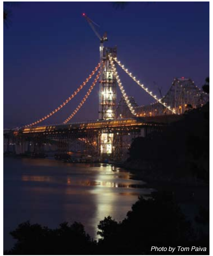
New lights on the East Span's SAS catwalks illuminate the path of the soon-to-be installed main cable that will support the decks.
