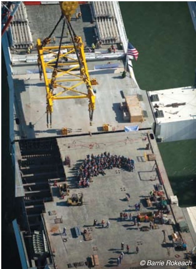
After the operation, the ironworkers gather to mark the completion of the East Span decks.
