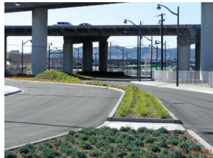
Permeable landscaped surfaces like the Mission Bay Circle will ease the strain on The City’s combined sewer system during heavy rains by absorbing water that would otherwise flow into the sewers.
