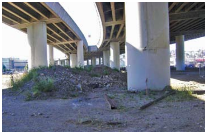
Mission Bay used to be cut off from its neighbor, the Potrero district, by the I-280 Freeway and a set of Caltrain tracks, with 16th Street providing the only access to the area from the west. But a new road opening in early-to-mid 2012 will provide another way to get to Mission Bay from 7th Street, via the landscaped Mission Bay Circle turnaround.
