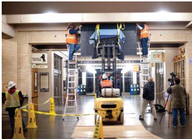
The 700-pound flap sign, which is eight feet wide, was installed in the Great Nave of the Ferry Building under the cover of night to avoid interfering with approximately 11,000 daily commuters and visitors.
