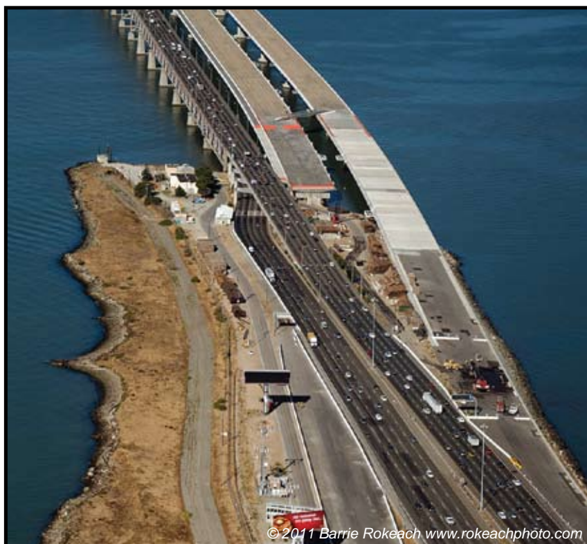
The Bay Bridge touchdown as it now exists, with the twin decks of the new East Span coming in from the right
