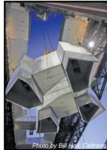
Photo by Bill Hall, Caltrans An underneath view of the grillage piece as it rises between the twin decks of the East Span
