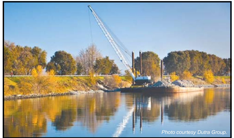
Strengthening Delta levees with rock from Dutra's San Rafael Quarry.
