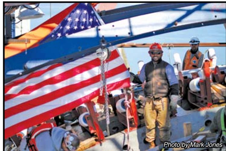
Workers attached an American flag to the final strand of the new bridge's main cable for its nearly mile-long voyage from anchorage to anchorage.
