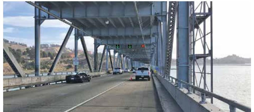
A series of newly-installed electronic signs indicates to motorists when the new third lane is open to traffic. Green arrows indicate open lanes and a red X indicates a closed lane.
